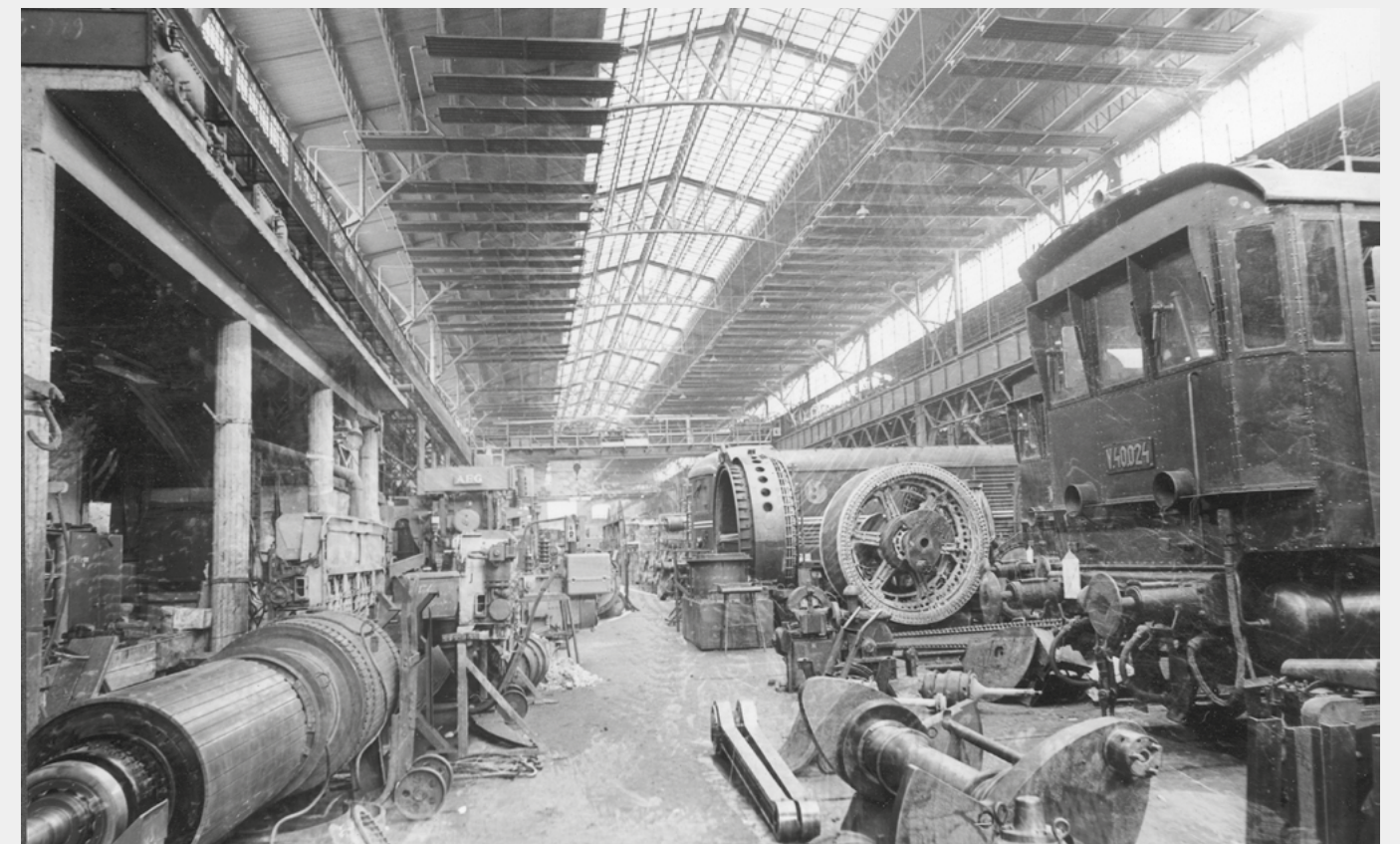
Figure 7 – The Eiffel Hall in 1965, at the time of the new ceiling radiation heating construction. Two V40 engines and one V55-type locomotive are being repaired in the hall; spare parts of their large-size electric equipment can be seen around the locomotives. (MÁV Archives, 518a)
